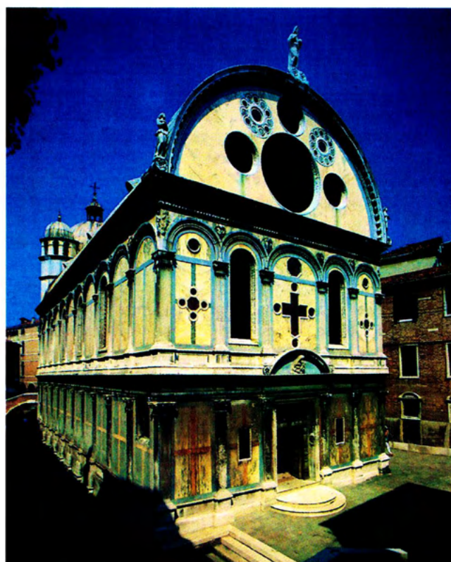
Fig. 1 - On the façade of the Santa Maria dei Miracoli church a strong decay due to atmospheric pollution was visible.
