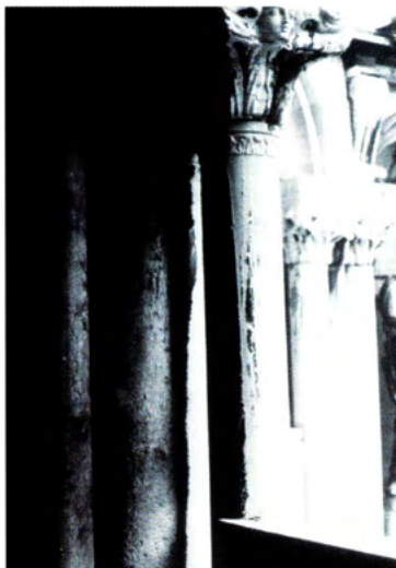
Fig. 17 - Black crusts occurred on sheltered areas from direct rainfall and are mainly formed by gypsum.
