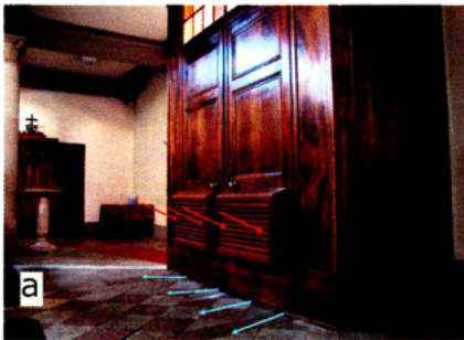
Fig.4 - (a) The main door is provided with two series of slits to allow the exhaust of internal air. Red arrows indicate internal air going out and blue ones external air leakage. (b) Infrared image of the door and the cold wall of the counterfacade. (c) Detail of the door slits and in/out air leakages.
