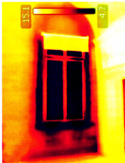
Fig. 6 - Water percolation. The portion of wall below the window has been moistened by rainwater percolated inside. Moisture has increased wall conductivity and lowered the thermal level of the indoor moist surface. The different conductivity between damp mortar and bricks makes the internal structure of the wall visible.
