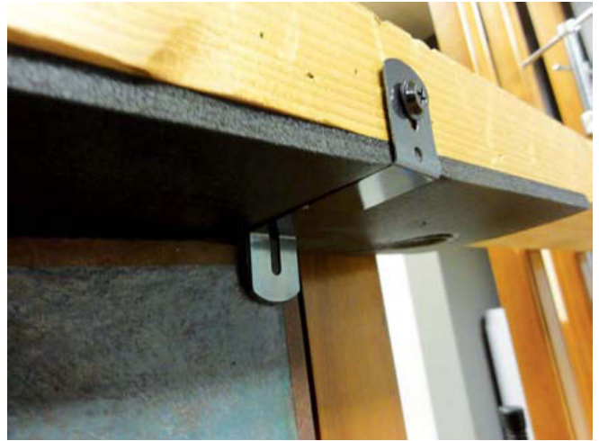
Fig. 10 – Screw padded mending plates into the top 2 x 4 so it lightly touches the face of the painting along the top edge preventing the painting from falling forward.
