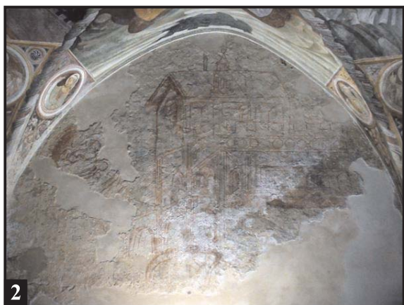
Fig. 2 – Chapel of Saint Biagio, sinopia remained in sight after the fall of the painted plaster
