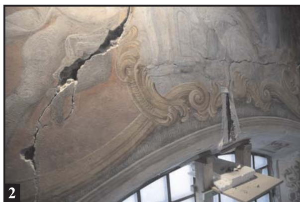
Fig. 2 – Removing of the old reparation.
